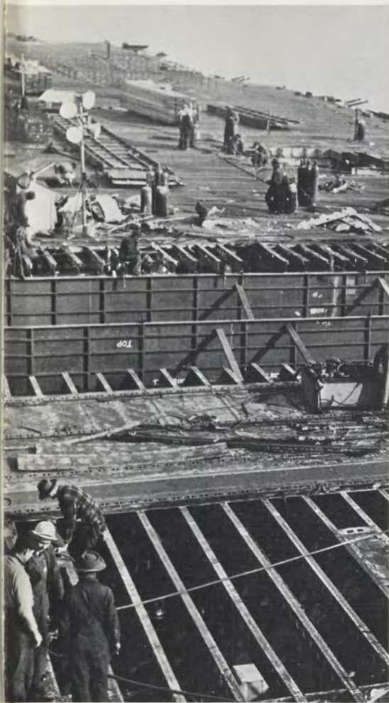
six days before the japanese attacked pearl harbor dec 7, 1941 the keel of uss intrepid (cv-11) was laid in a concrete graving dock at newport news, va. seventeen months later a 44 million dollar aircraft carrier the length of three football fields stood ready for her initial plunge.
