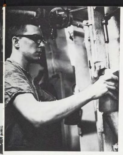
Drawing water from a boiler for sample testing
