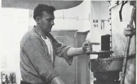
Cutting steam from the boiler into the steam system of the ship
