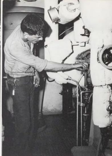
Adjusting make-up feedwater within the main boiler feed system
