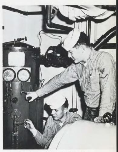
Lube Oil Filter in Operation
