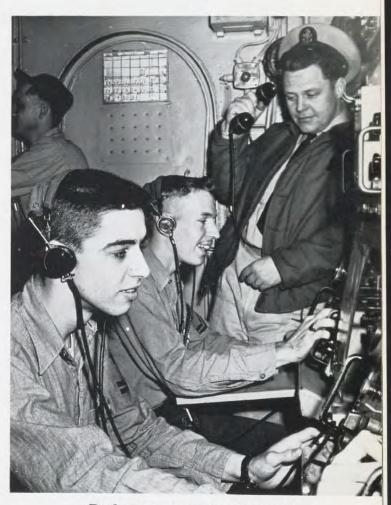
Radarmen operate electronics counter measure equipment
