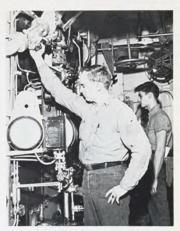
This man checks feed water supply to boilers
