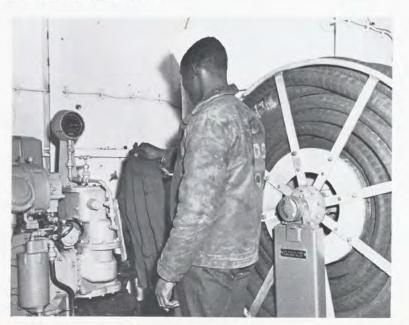
Aircraft Fuel Pump Being Checked
